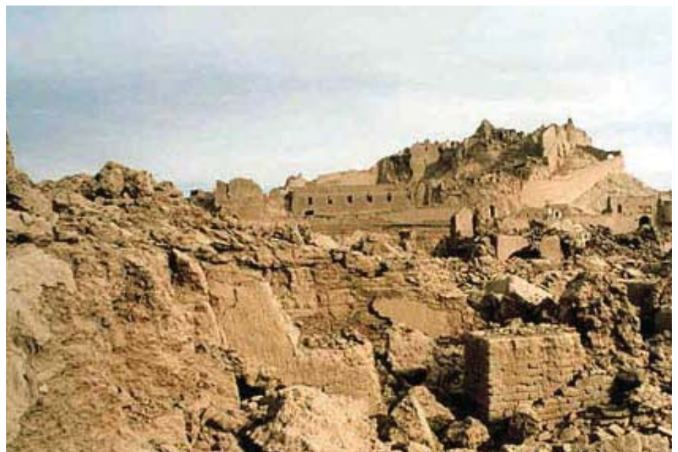
After earthquake: Walls believes that devastated citadel and city can be reconstructed.
