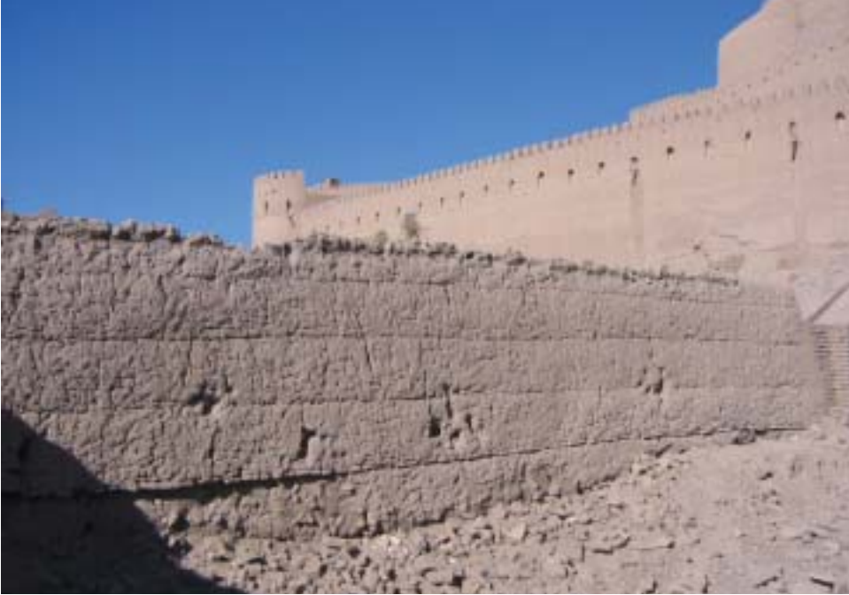
Layered mud-brick construction which, claims Walls, is more resistant to earthquakes than modern cement mixtures.
