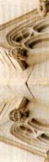
The projecting gargoyles were severely eroded and the rest masonry had to be cut out and totally replaced.
